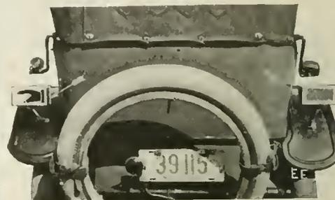
You Can't Miss this Electric Auto Indicator. The Illuminated Hand at Right or Left indicates Which Direction the Machine Is Going to Take. Works in Daytime as Well as Night.
