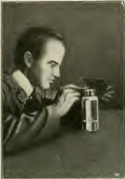
Fig. 89. Interesting Experiment with Sodium and Water. The Lighted Splint or Combustion Test is Tried After the Sodium Has Been Dropt in the Water.
