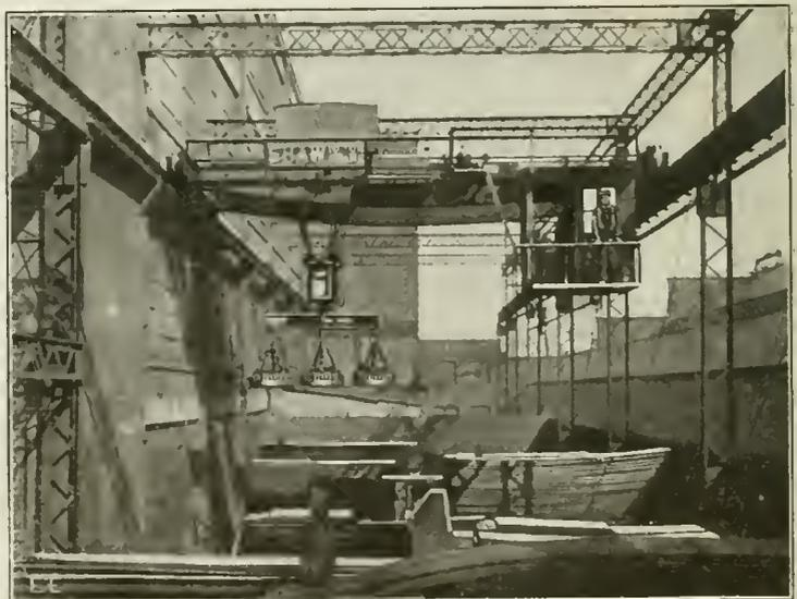
To Reduce to a Minimum the Cost of Labor in Handling Steel and Iron Plates, an Ohio Plant Utilizes Three Large Electro-Magnets Suspended From a Swiveling Beam Carried by a Travelling Crane. The Plates Can Be Released in Any Position.
